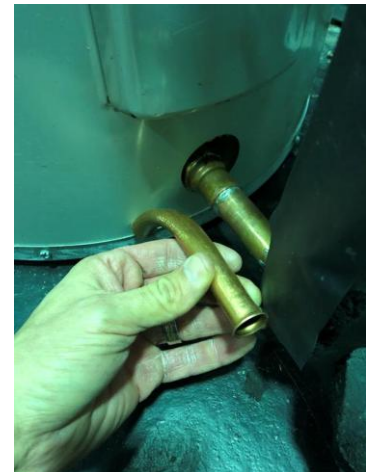
Figure 81: Retrofit Dispersion Tube fabricated from \frac{1}{2} " Copper Tubing
