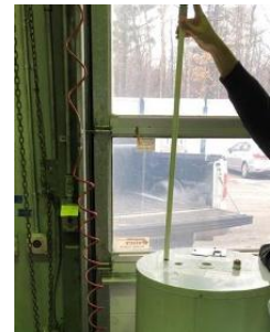
Figure 78 Removing the Dip-Tube from the tank
