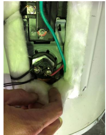
Figure 83: Removing the Bottom Access Cover to expose the Storage Tank Surface and Lower Heating Element Wiring
