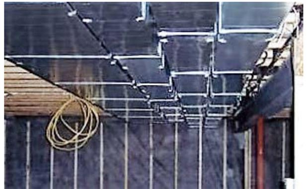
**Figure 5-7:** Three Rectangular Zone Supply Trunks, with the Return Trunk shown on the Left
