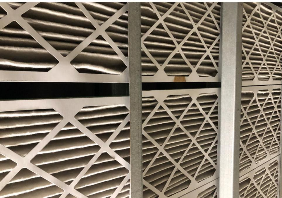
Example of filter rack assembly allowing significant air flow bypass
