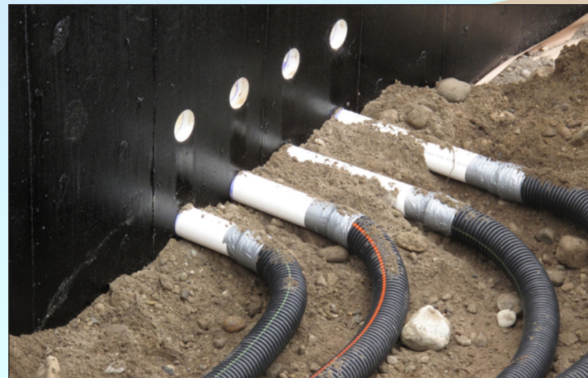
Figure 3. Watertight connection of tubes to a building
