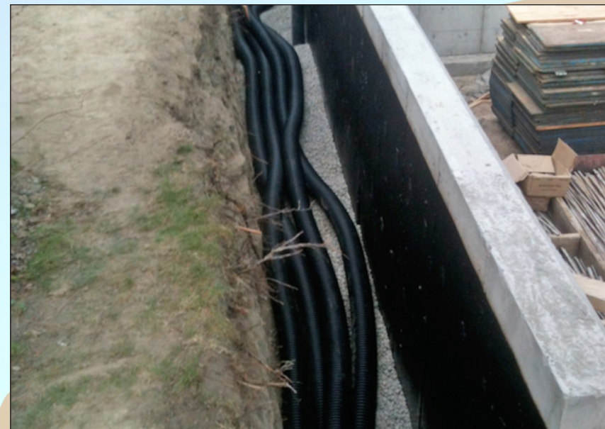
Figure 3. Pipes in a trench before it is backfilled
