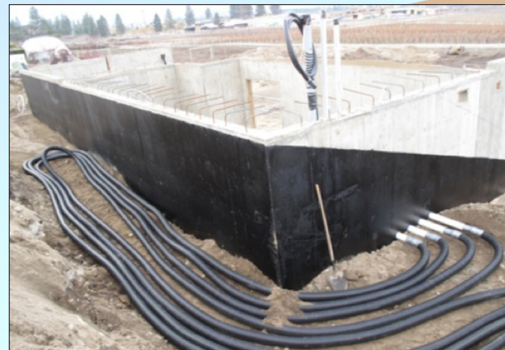
Figure 1. The layout of tubes with lower layer already backfilled
