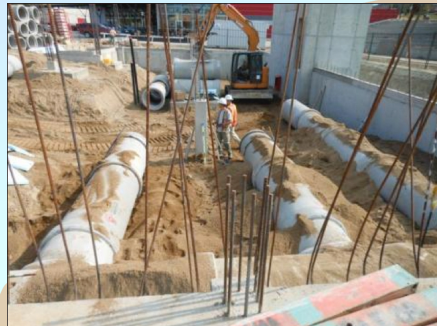
Figure 3. Pipes in a trench before it is backfilled.
