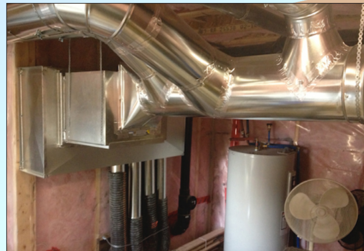
Figure 1. The layout of tubes connected to a supply fan and ducting.
