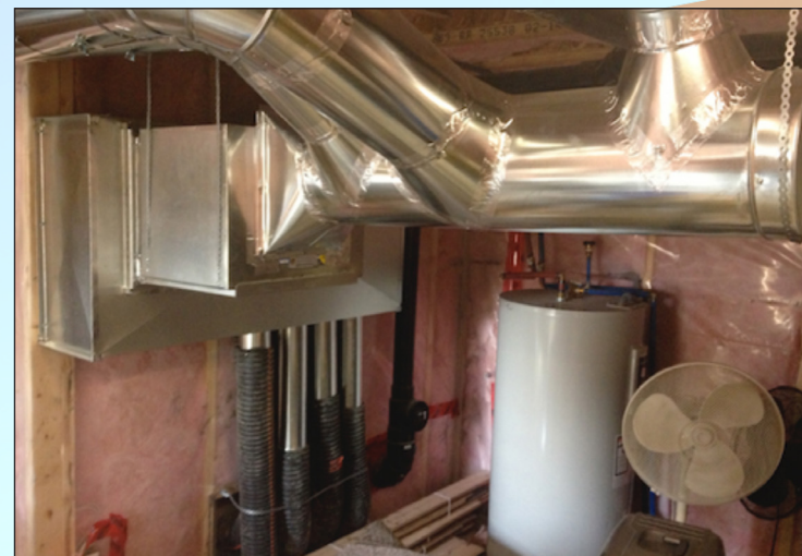
Figure 1. Layout of tubes connected to a supply fan and ducting
