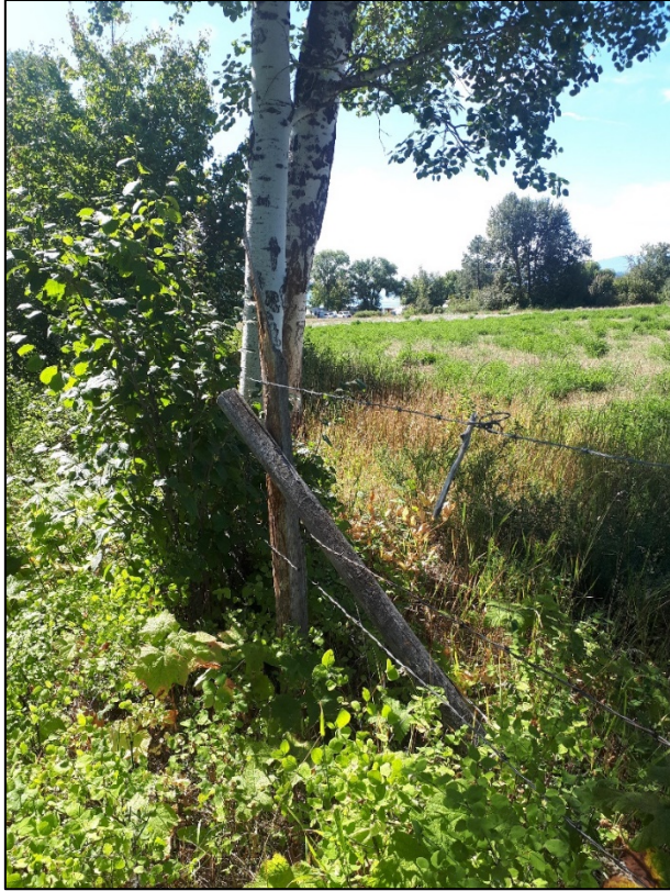
Image 12: Southwestern fence line in Lot 79 showing growth of poplar trees into fence posts and old posts taken on 29 August 2019.
