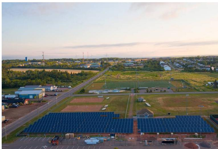
**Figure 2:** Credit Union Place Smart Solar Storage System with 494 kW<sub>p</sub> array in Summerside, Prince Edward Island.
