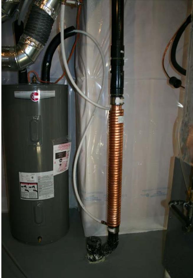
Figure 21: Installed Drain Water Heat Recovery system in LEEP field trial home.
