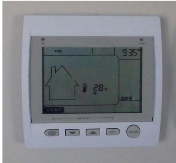
**Figure 20: Image of an installed advanced controller in a LEEP field trial home.**
