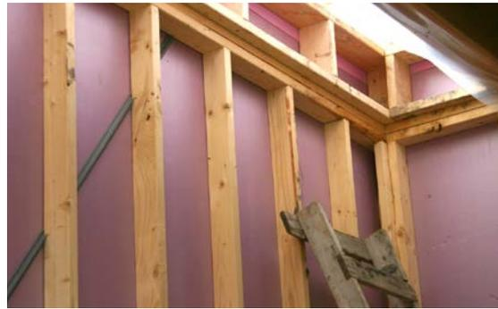
**Figure 8:** Rigid foam insulation system used in Winnipeg trial home to replace exterior wood sheathing as well as the air barrier, 2015.
