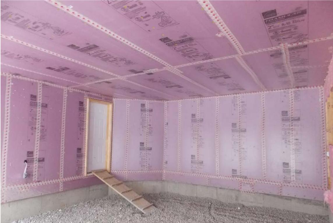
**Figure 14: Example of foam board sheathing applied to the underside of a floor above a garage.**
