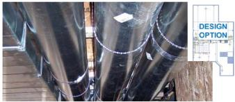
Figure 5-8: Three Round Zone Supply Trunks, with the Return Trunk shown on the Left
