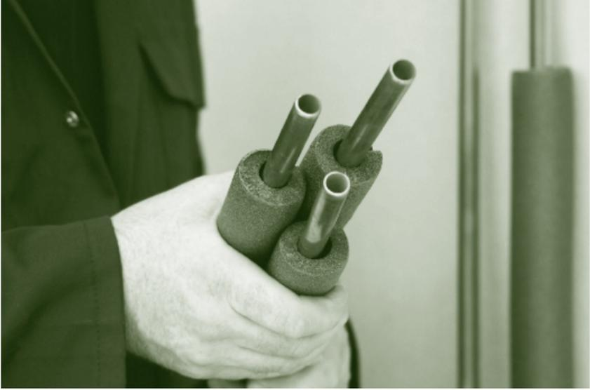
Insulating the hot and cold water pipes within 2 to 3 m of the water heater is the most cost effective improvement that can be made to existing or new installations. Several products can do this job, but the easiest one to use is the pop-on insulating foam sleeves. They are very effective and can be mitred at bends in the pipe.
