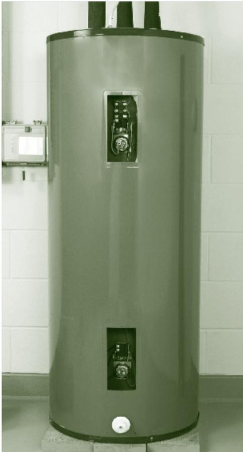
New water heaters must have a temperature and pressure relief valve. This safety device allows water that is too hot or under too much pressure due to a faulty temperature control to escape from the tank.
