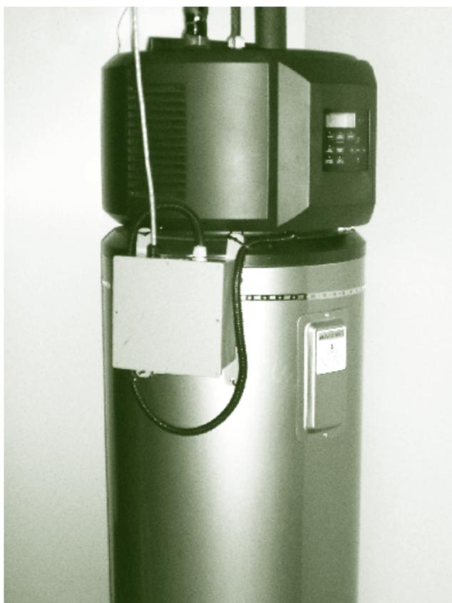
**Heat pump water heaters** (HPWHs) use electricity to transfer heat from the air instead of converting electricity directly to heat. Heat is taken from the air in the basement or utility room (or sometimes from outside) and transferred to a tank of water.
