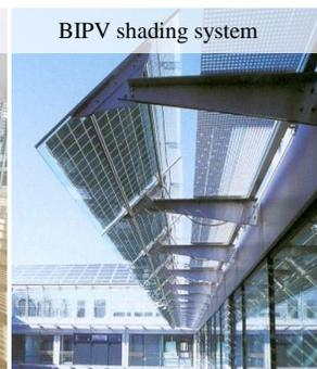
BIPV shading system
