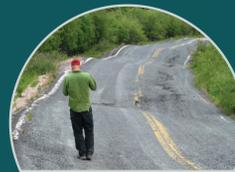
The frozen ground, called permafrost, in Canada's north is warming, which can cause the land to sink, damaging buildings, roads and other infrastructure.
