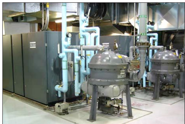
Photo: IBM. The Bromont plant replaced a vacuum system that used air compressors with a central vacuum system.
