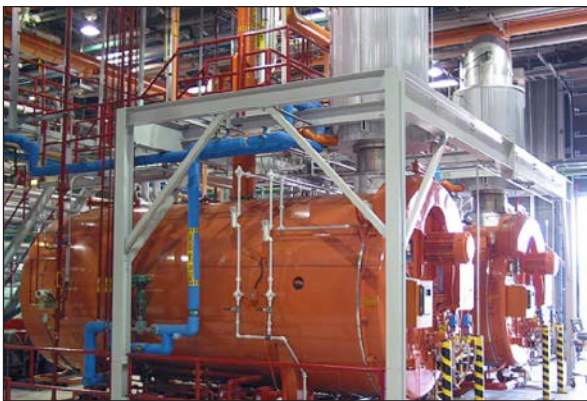
Photo: IBM. Four steam gas boilers (natural gas, oil backup): 73 000 lb./hr, 2200 hp, 50 to 125 psi. Enough energy to heat about 1000 average homes for one year. Used for heating, humidification and the production process.
