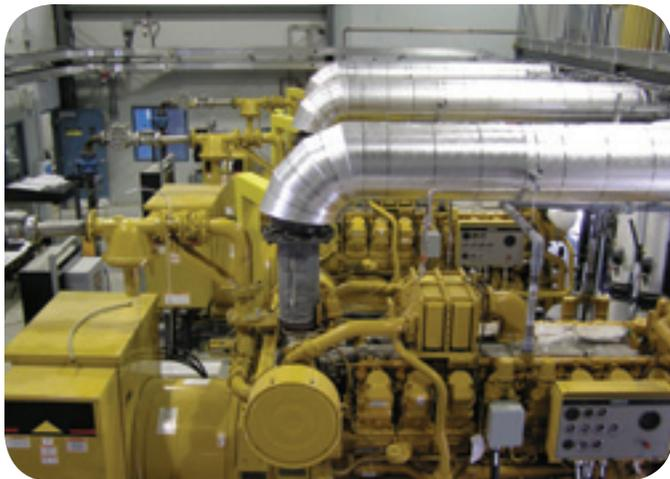
Electricity generated from landfill gas is sent to the grid. The use of waste heat in a nearby new development is under evaluation. (Ecotricity Guelph Inc., Guelph, Ontario)
