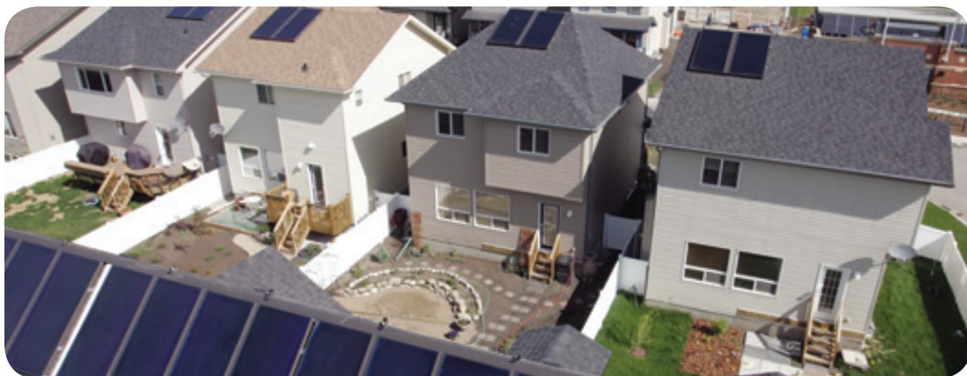
*Solar energy heats energy-efficient homes using solar thermal collectors, seasonal thermal storage and a district heating system. (Drake Landing Solar Community, Okotoks, Alberta)*
