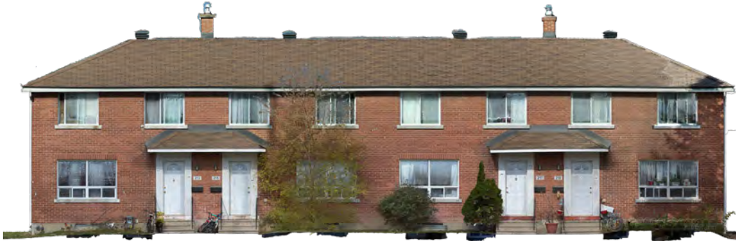
Figure 7-7: Scaled, measurable 2D ortho-elevations can be imported into CAD software
