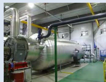
The Organic Rankine Cycle turbine and condenser unit at the Nechako Lumber Company in Vanderhoof, B.C.
